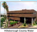
Hillsborough County Water Department Administration Building Hillsborough County, FL
